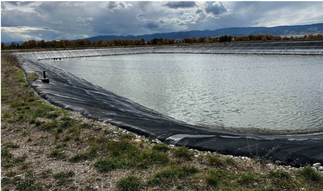
Figure 2-20 Treatment Lagoon Cell 1
